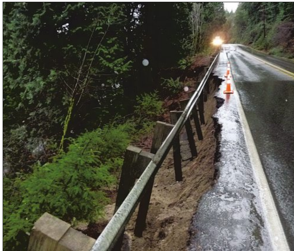
PHOTO COURTESY OF WASHINGTON STATE DEPARTMENT OF TRANSPORTATION
