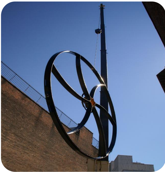
Assembled steel frame flying into position.
