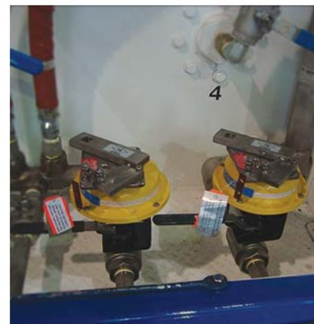
High pressure thermal shut-off assemblies for a compressed gas.
