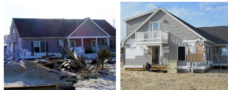
Damage caused by Hurricane Sandy
