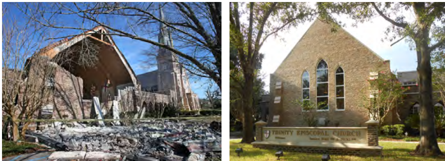
Left: Damage caused by tornado Right: Church rebuilt after tornado damage
