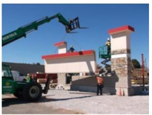
CUTLINE: Fullerton Building Systems' prefabricated building panels speed up construction time on new franchises.
