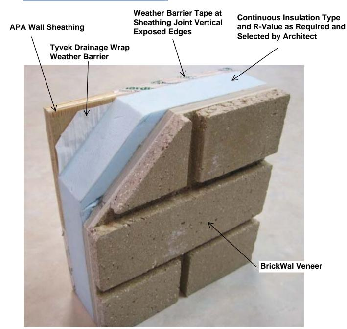
**Standard Detail With Countinuous Insulation Added**
