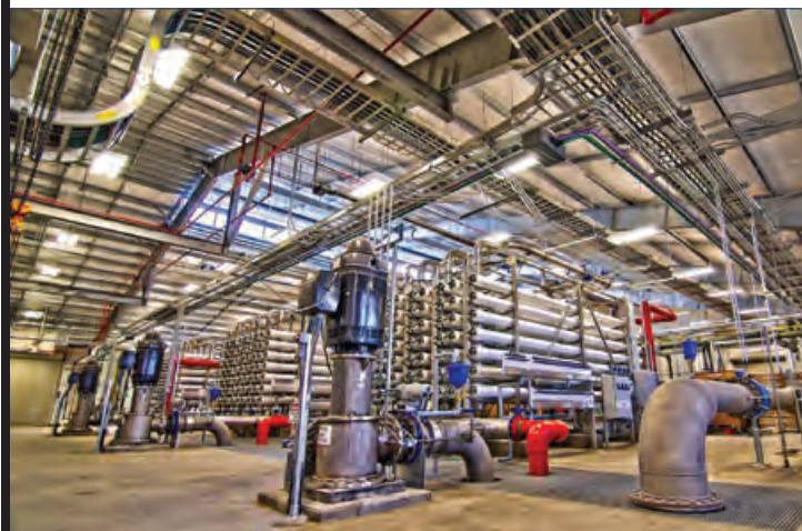
Hatch Mott MacDonald ( No. 36 ) designed a 9.6-mgd reverse-osmosis water treatment plant, coupled with EPA Class 1 deep-injection wells to dispose of uranium-contaminated brine, for the city of Sterling, Colo. ■
