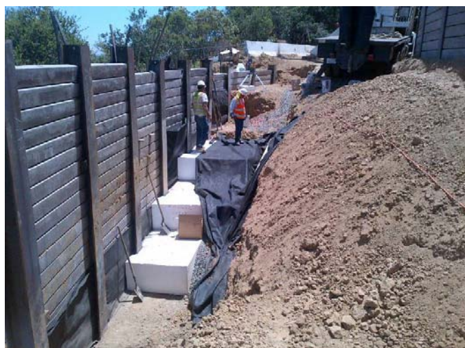
Figure 8. Light weight geofoam backfill is being placed behind the retaining wall at Station 176
