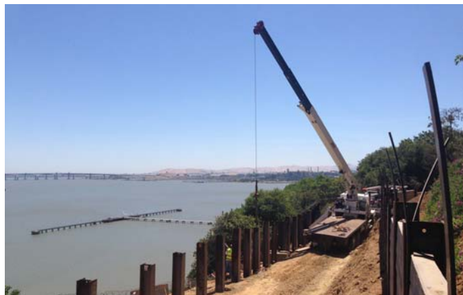
Figure 7. Installation of steel soldier piles at Station 176
