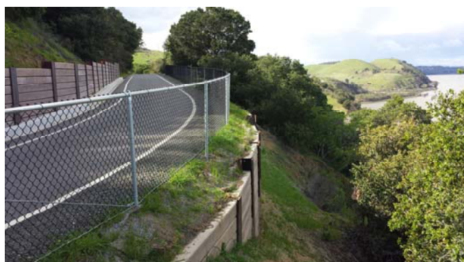
Figure 9. Completed retaining and debris walls at Station 176 (same view as Figure 5)
