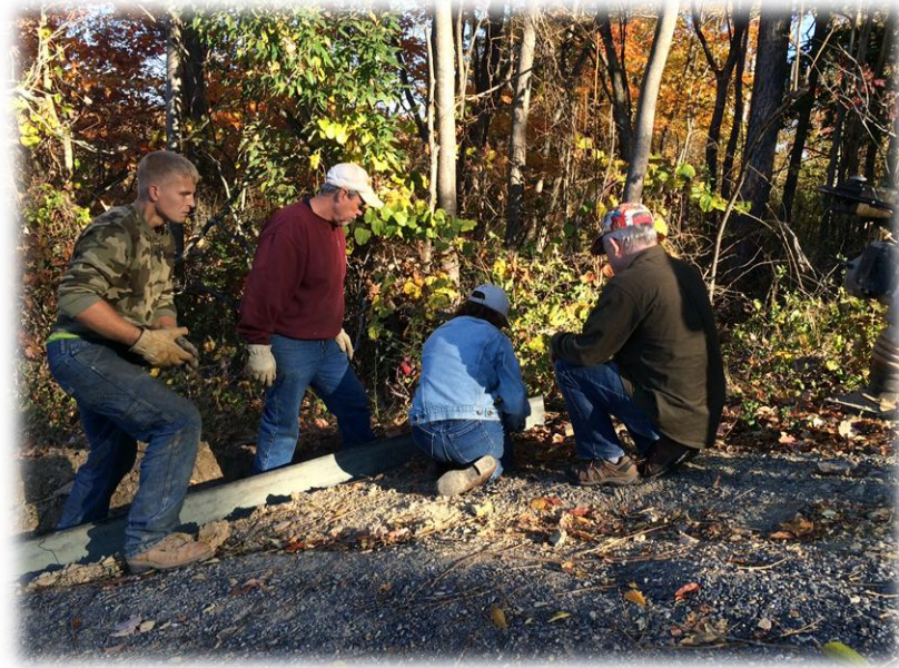
Installation of the water diverters
