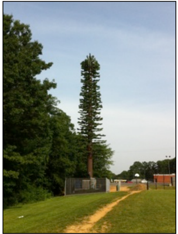
Completed treepole after branch installation
