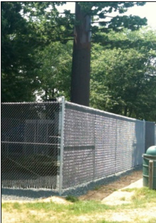
Fenced in equipment before landscaping.
