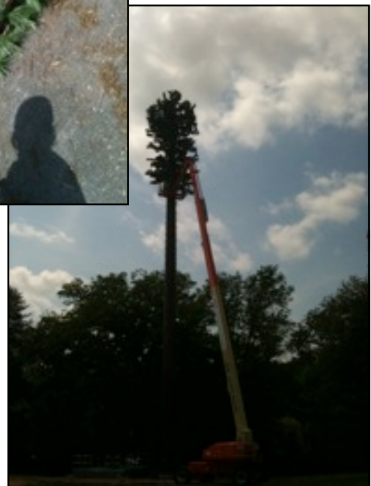
Branches are attached by a technician suspended by a crane.
