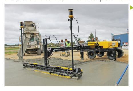
creeding is the process in which a concrete finisher cuts off excess wet concrete to bring the top surface of a slab to the proper grade and smoothness. Traditionally, concrete contractors can perform this task using a flat board or an aluminum tool after the concrete has been placed. Through the years however, technology has improved the process and many contractors are experiencing positive impacts on labor and material costs while also increasing profits.
