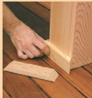
Assemble base moulding
