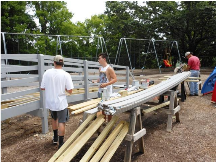
The ramp that makes the playground handicapped accessible is being rerouted and upgraded with boards that won't have splinters or need painting.
