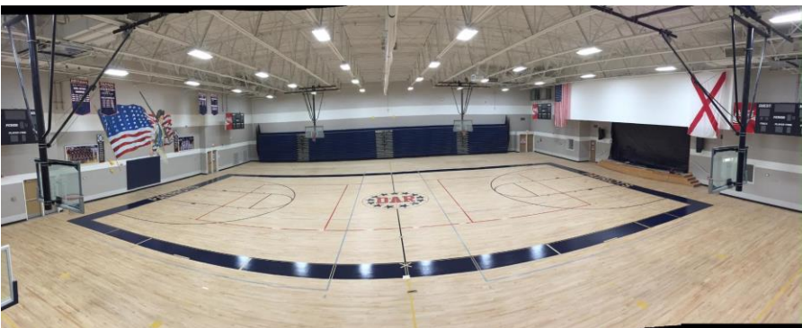
The finish on the gym floor of the Burkey Center was sanded down to the bare wood and refinished with a new paint scheme and lines.
