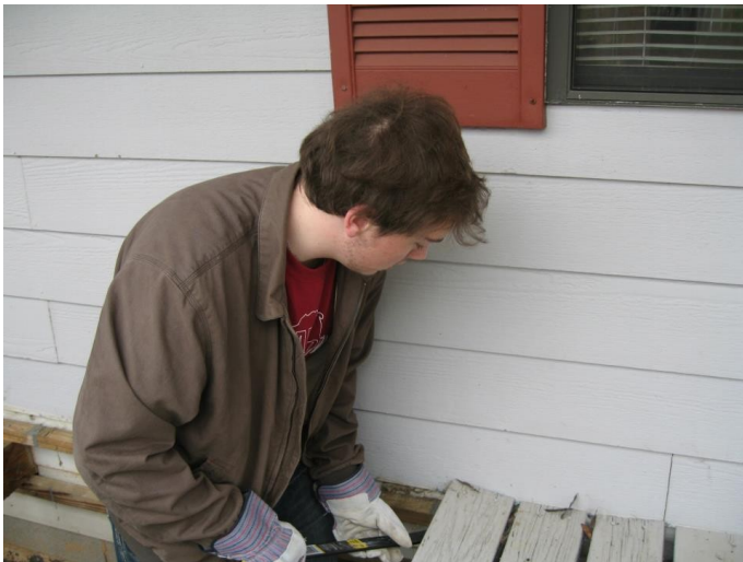
Hank Selby prys up old wood with a crowbar.
