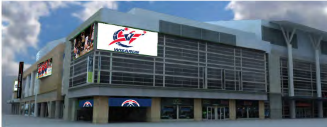
View from 7th Street NW and F Street NW looking north.
