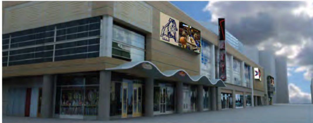
View from 7th Street NW looking south.
