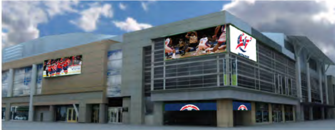
View from 7th Street NW and F Street NW looking northeast.
