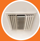
Air and duct sealing
