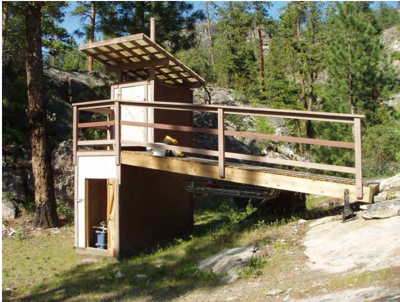
Plate 18: The composting toilet located within a high use climbing area of the park.
