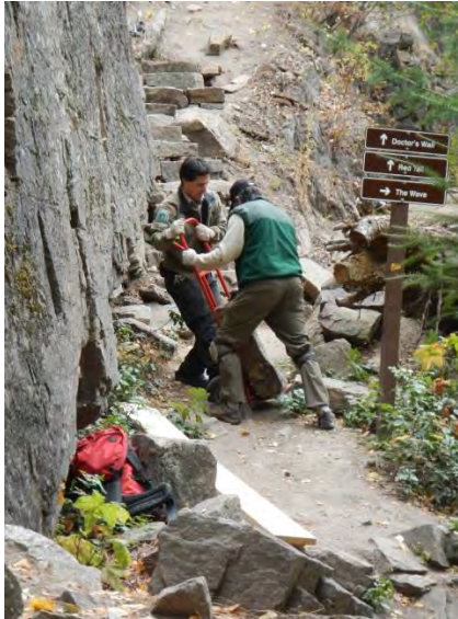
Plate 17: Parks staff extending the rock stairs along the Red Tail trail.
