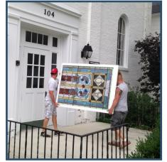
After the restoration is completed the windows are returned to the Seminary Building. The windows are re-installed and a covering of tempered glass is added to the exterior of the window for maximum protection. The next two windows are then removed for transport to the studio and the process continues.
