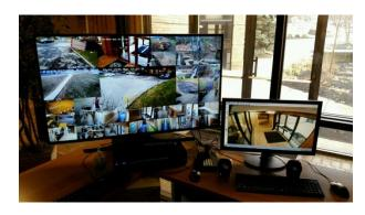
The camera system at CTA has been replaced to enhance security and safety monitoring both inside and outside the walls of our building. Evaluation of our old system showed a 15 to 20 year old system with mostly analog cameras. Only 10 out of the 30 cameras were operational and the recording features were basically not usable.
