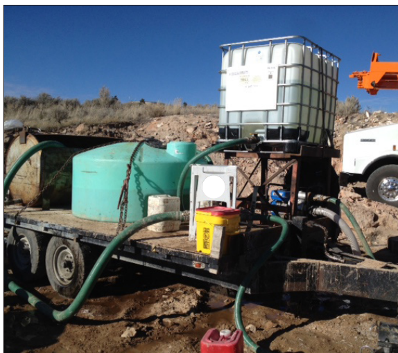
Figure 2: Mix tank and Injection tank set up
