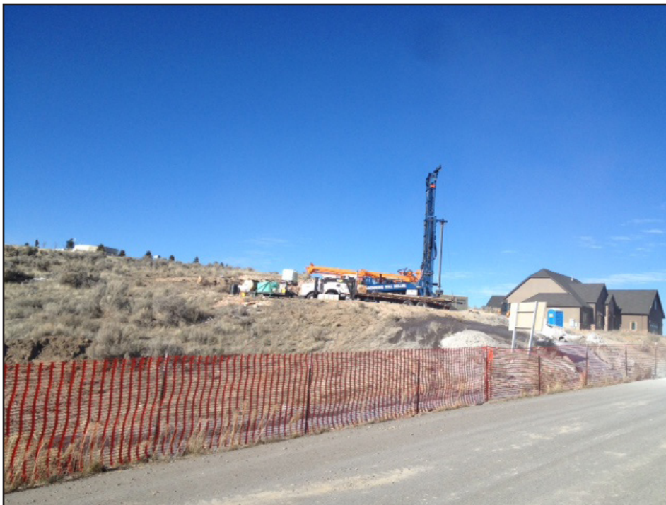
Figure 1: Drill location and set up
