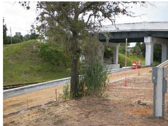
10<sup>th</sup> Street (SR 17) Improvements Project is a 1.5 miles roadway reconstruction and utilities installation project from Scenic Highway (SR 544) to Hinson Avenue (US 17/92). The project includes new curb and gutter, sidewalks, lighting, storm drain modifications, gravity sewer, force main and water main. Currently, the project is 90% complete with an anticipated completion in September 2015.
