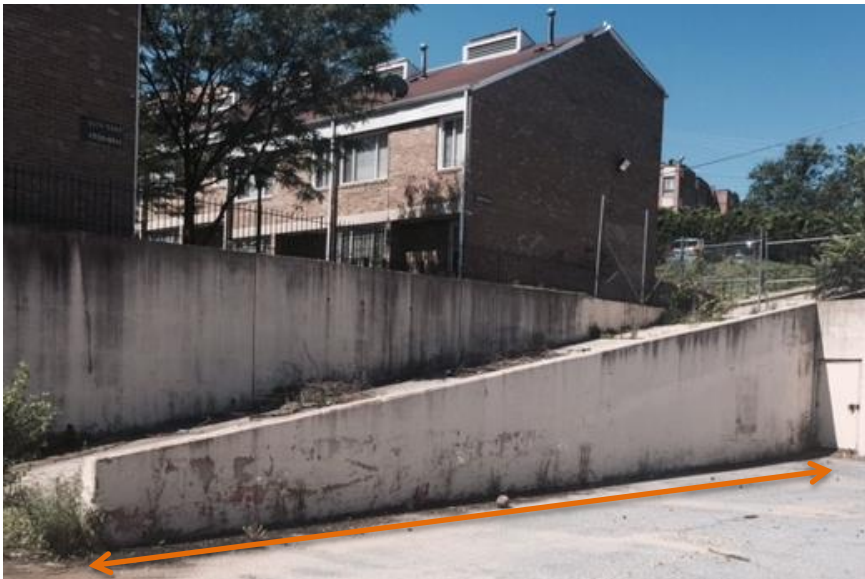
Wall 1 (lower wall) – dimensions: 57' long x 12' tall at highest point
