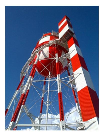
Tower. In order to keep the tower functioning for port operations, it needed to be repaired. To mitigate corrosion damage in the future and to restore the tower to its original orange and white color scheme, a new coating system was included in the restoration project.
