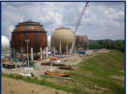
All sphere welds were 100% Ultrasonic Tested (UT) in lieu of radiography as allowed by ASME Section VIII.
