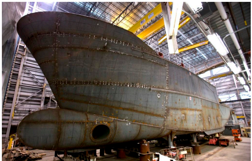
Construction of the 136' F/V Arctic Prowler in Ketchikan, Alaska.
