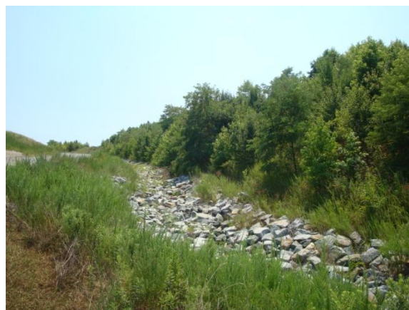
Existing riprap lined stormwater channel before start of project.
