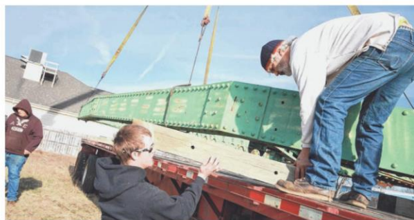
Jordan Curtis helps Nels Raynor put large pieces of wood under a piece of the Indian Trail Bridge. It will help keep the piece in place as a truck drives it to Purdue University in West Lafayette, Ind., this week.
