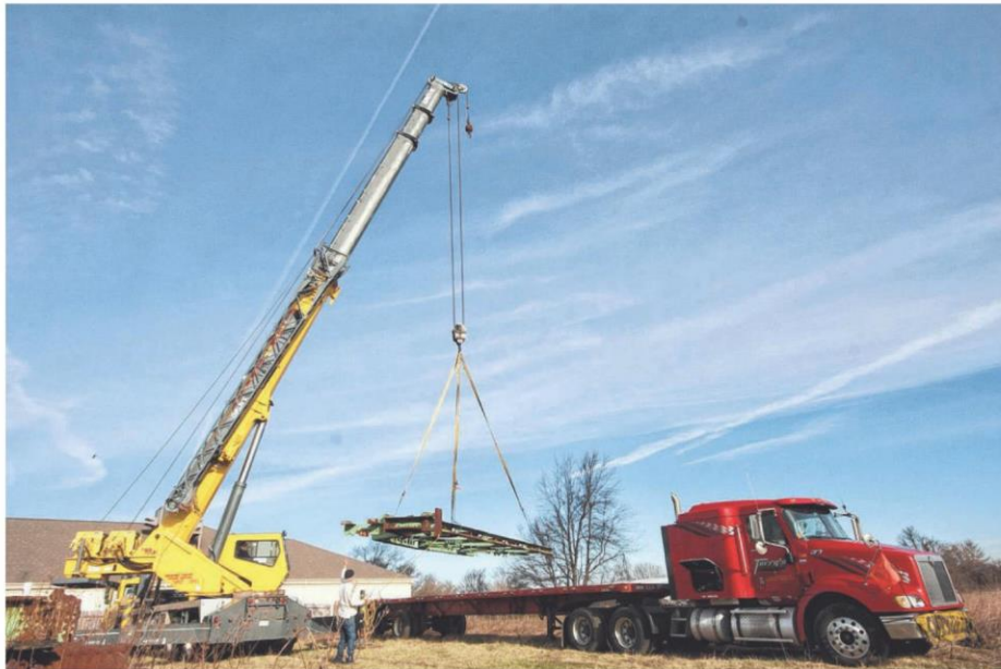
Crane operator Leo Schnieder and Nels Raynor of Back Ornamental Iron work together Wednesday morning in Marshall to load parts of the Indian Trail Bridge onto a truck. It will be transported to Purdue University in West Lafayette, Ind., this week.
