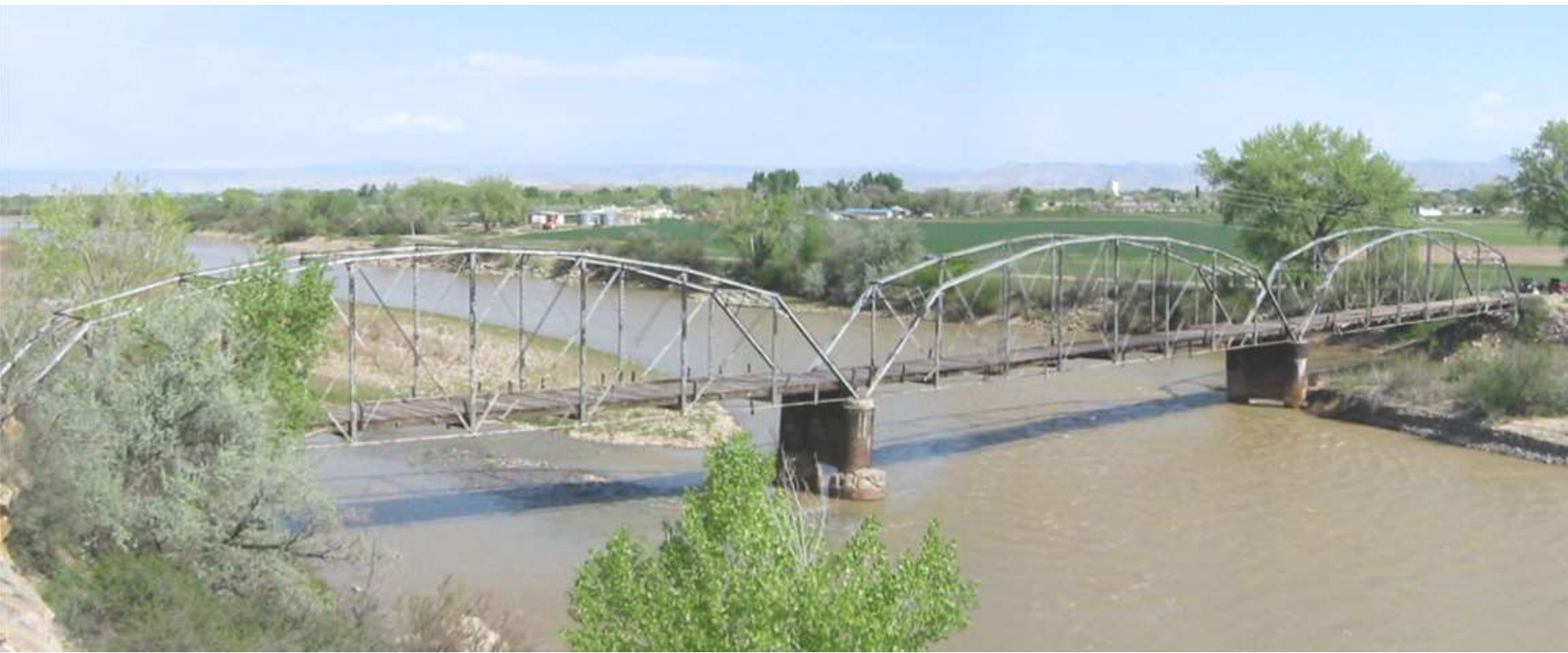
Fruita Bridge over Colorado River
