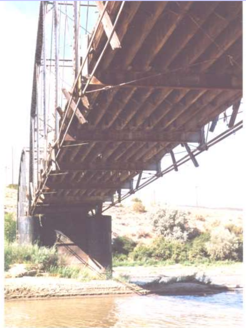
Fruita Bridge Underside
