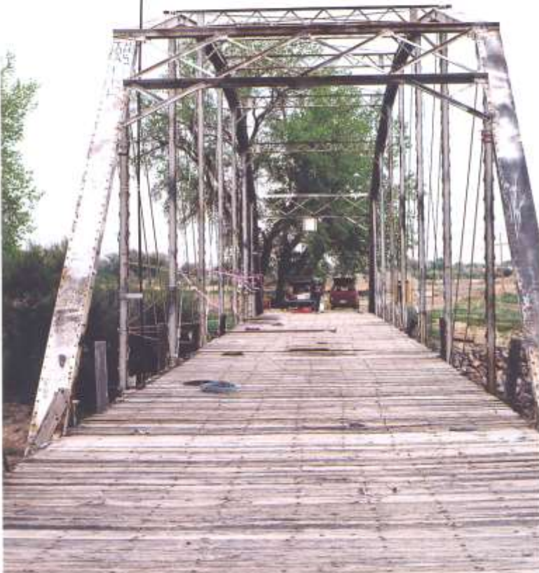
Fruita Bridge Deck
