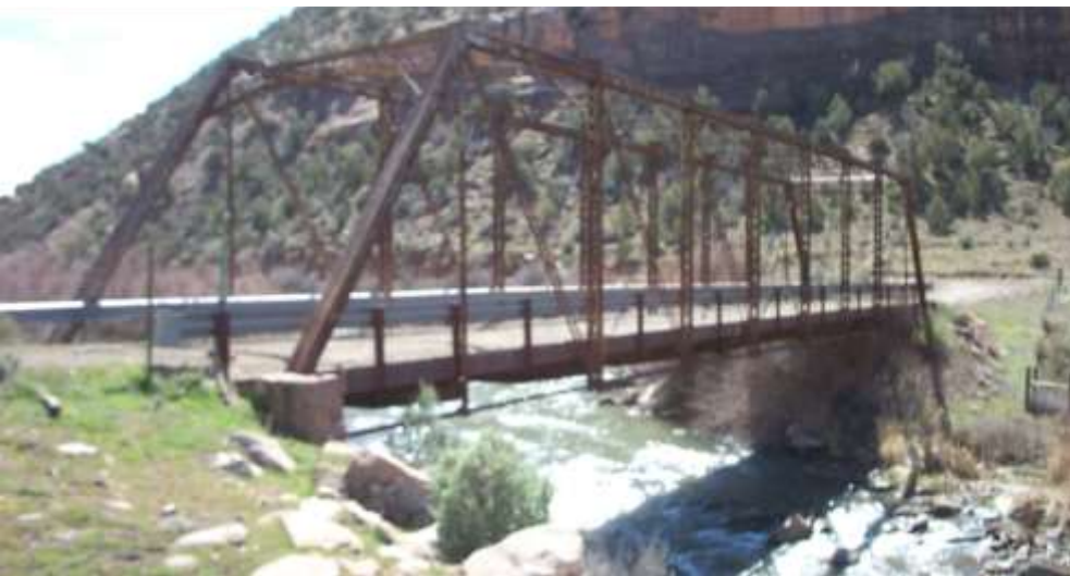
San Miguel Bridge Uravan, Colorado
