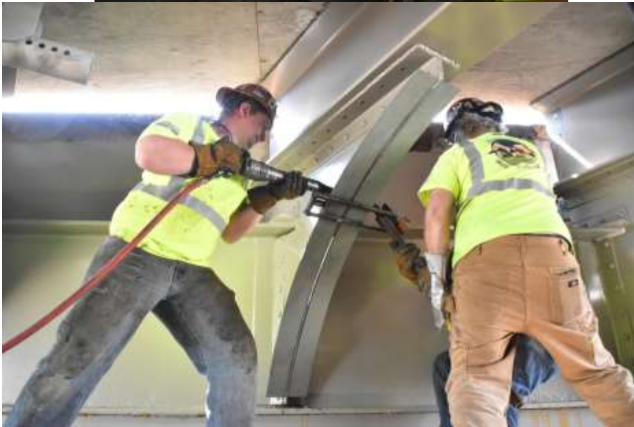
M-72 Bridge Hot Riveting In The Field (Tight Locations)
