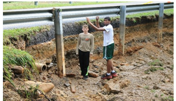
Flood waters eroded the road leaving guard rails damaged.
