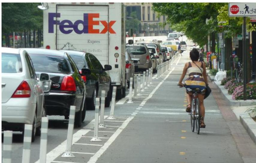
*The 15<sup>th</sup> Street Cycletrack in Washington, D.C. (above) is similar to the planned cycletrack for Baltimore where Parked vehicles (left) and a striped buffer (center) provide cyclists 2 layers of separation from moving traffic.*
