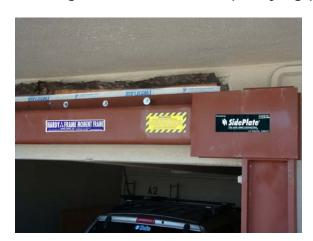
in the construction industry that enable contractors to buy standardized, locally available products to retrofit soft-story structures with at the least cost with the minimum disruption to the residents and with the best results to strengthen the
